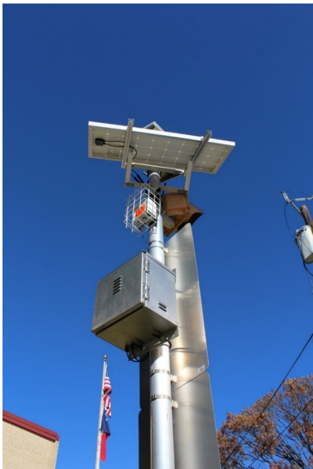
Figure 3: AQY1 Installed in Dallas.
